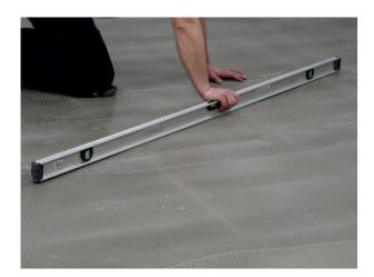
levelling compound, and a check must be carried out to determine if a sealer is needed.
