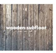
spiral Gluedown cannot be installed on most wooden substrates without special preparation. Either specific levelling compounds must be used, or the wood subfloor must be covered with special layers, e.g. plywood panels. These panels must be firmly attached to each other/the wood substrate and/or be glued or fixed. If there is moisture in the wood-based subfloor or there is no proper moisture barrier below the wood-based subfloor, it has to be removed first.
