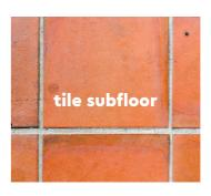
SPIRIT Gluedown can only be installed on top of firmly levelled subfloor for all gaps between ceramic tiles will telegraph through. Installation directly on unlevelled top of ceramic tiles is not recommended!
